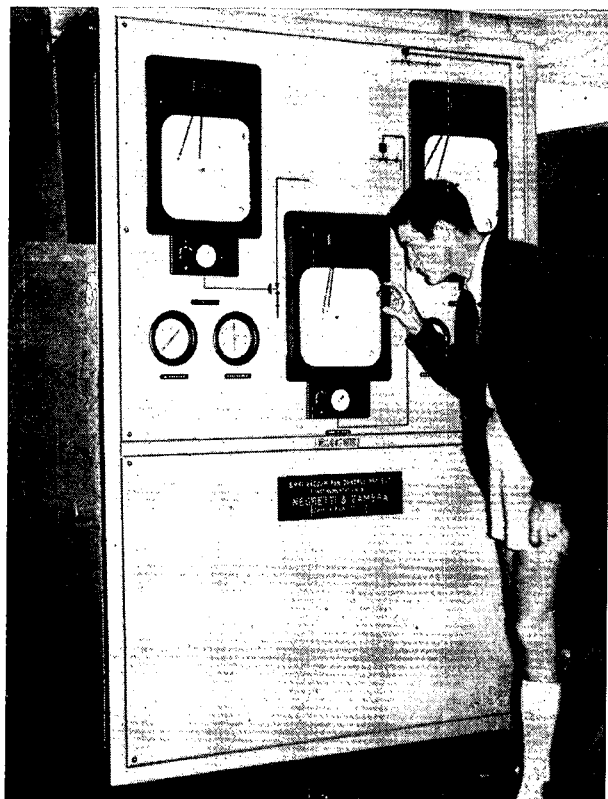
FIGURE 4: Control Panel showing Vacuum, Steam and Syrup Feed Controllers together with ancillary gauges
