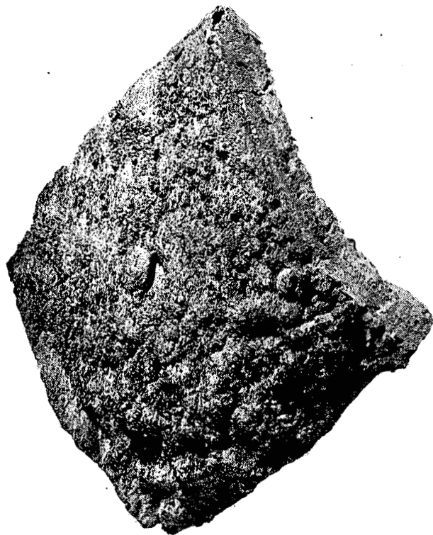
A: Deposit taken from generating tube showing heavy build-up causing chokeage through birdnesting. Chord dimension 4".
