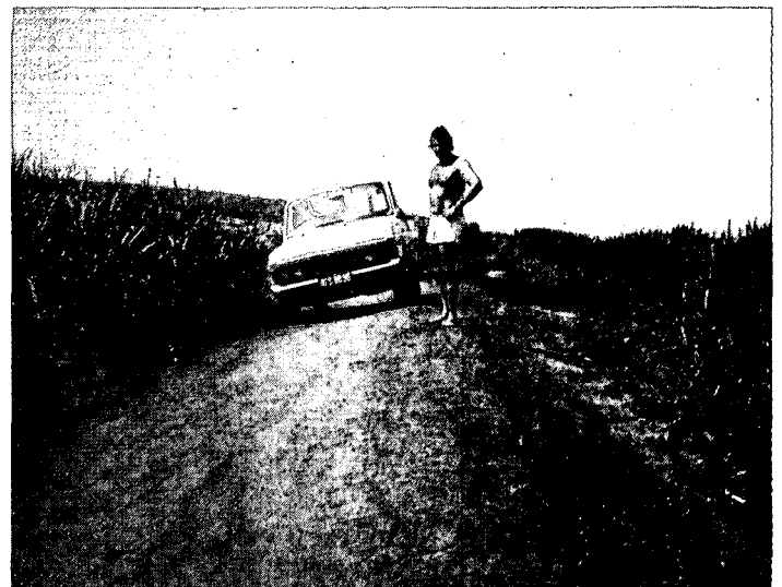
FIGURE 11 Terrace road showing the backslope into the hillside and the waterbearing channel.
