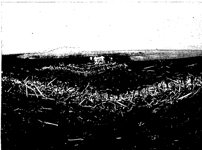
FIGURE 9 View of newly constructed waterway, showing cane top revettes.
