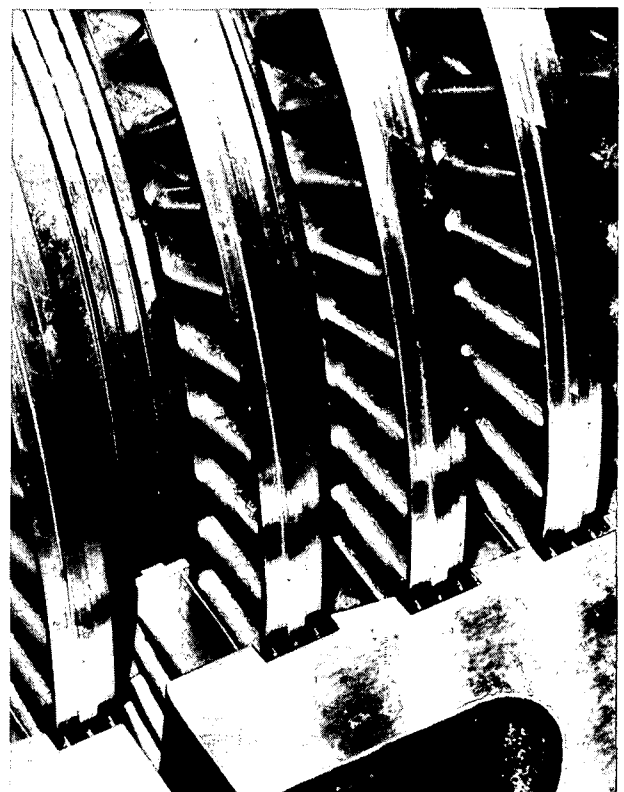
FIGURE 5 View of the Rotor- and Stator Blades.
