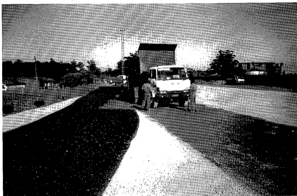
Figure 3. Application of bitumen chip and spray over polymer stabilised base in Experiment 19.
