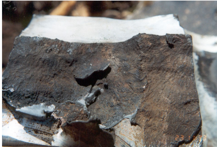
Figure 2. Corrosion fatigue in a steam drum.
