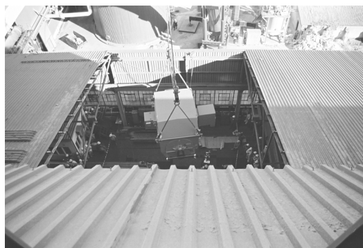
The new alternator being lowered through the power station roof
