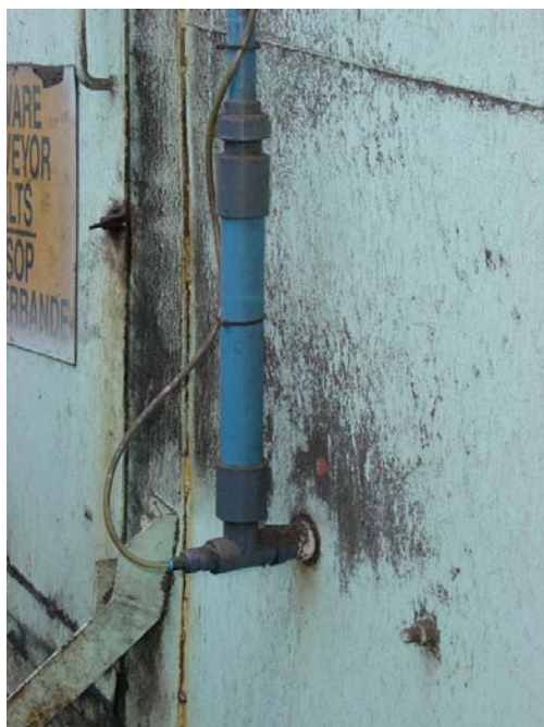
Figure 3. Solids trap.
