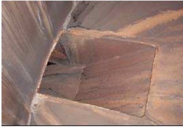
Figure 4. Unmodified injection water trough.
