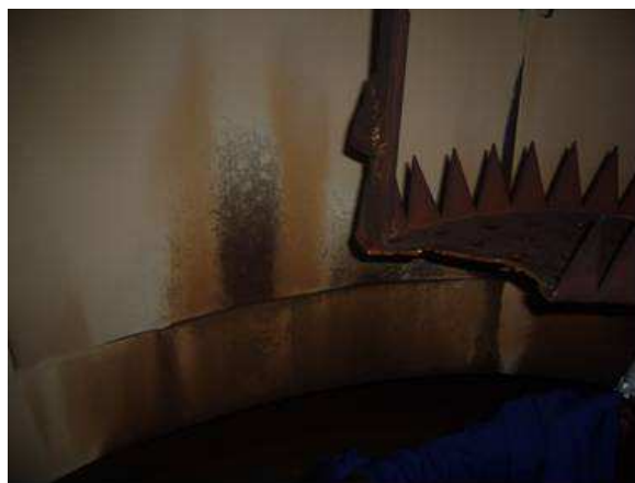
Figure 4. Broken section of the condenser rainmaker.
