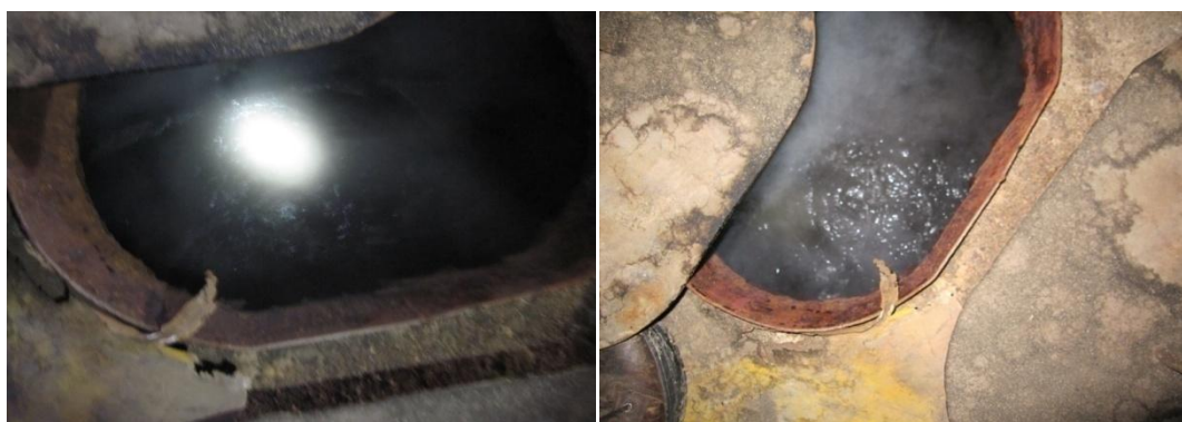
Figure 8. Surface conditions in the different hatches of the retrofitted clarifier.
