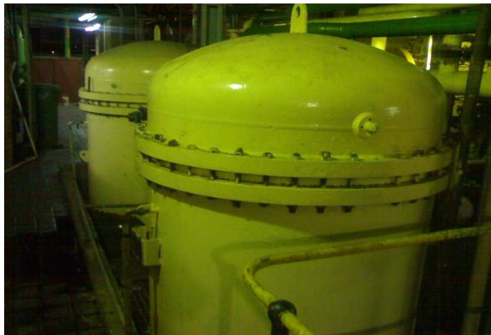
Figure 3. Polish candle filter at Pongola.
