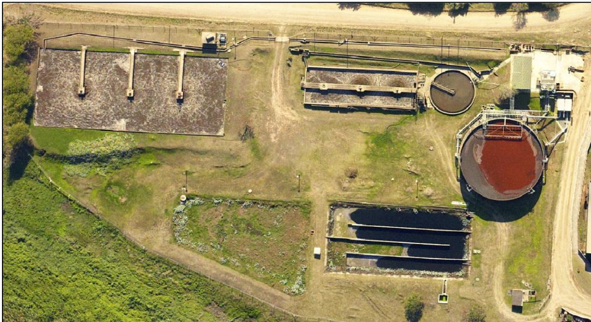
Figure 3. Aerial view of the effluent treatment plants at Sezela.
