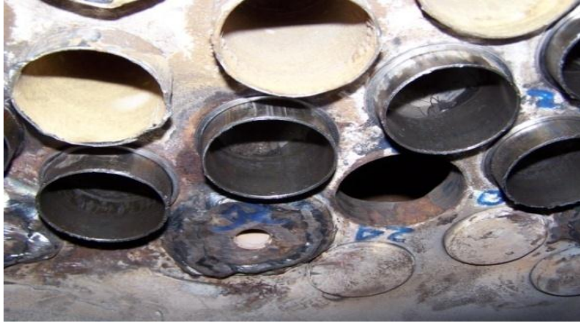
Figure 6. Tube plate holes after sleeving.
